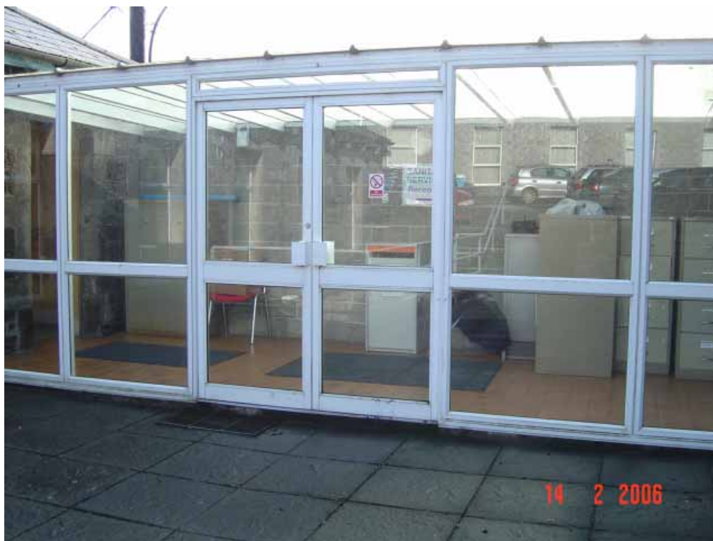
Fig 4.3 Entrance must be contrasted and small ramp installed to make this office accessible to all.
