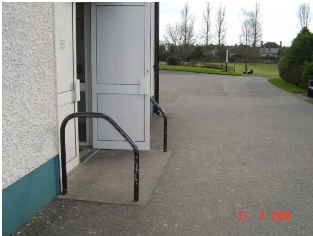
Fig 14.1 Identifiable level entrance.
