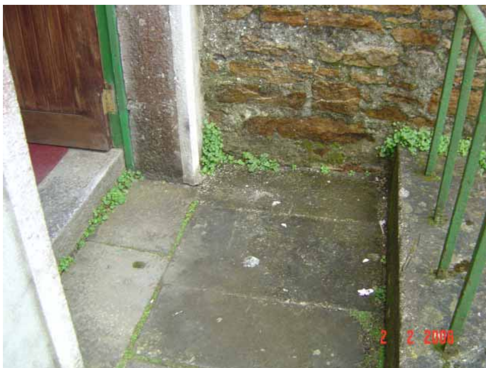
Fig 8.5 Existing doorstep with little room for manoeuvre and also 120mm entrance step.
