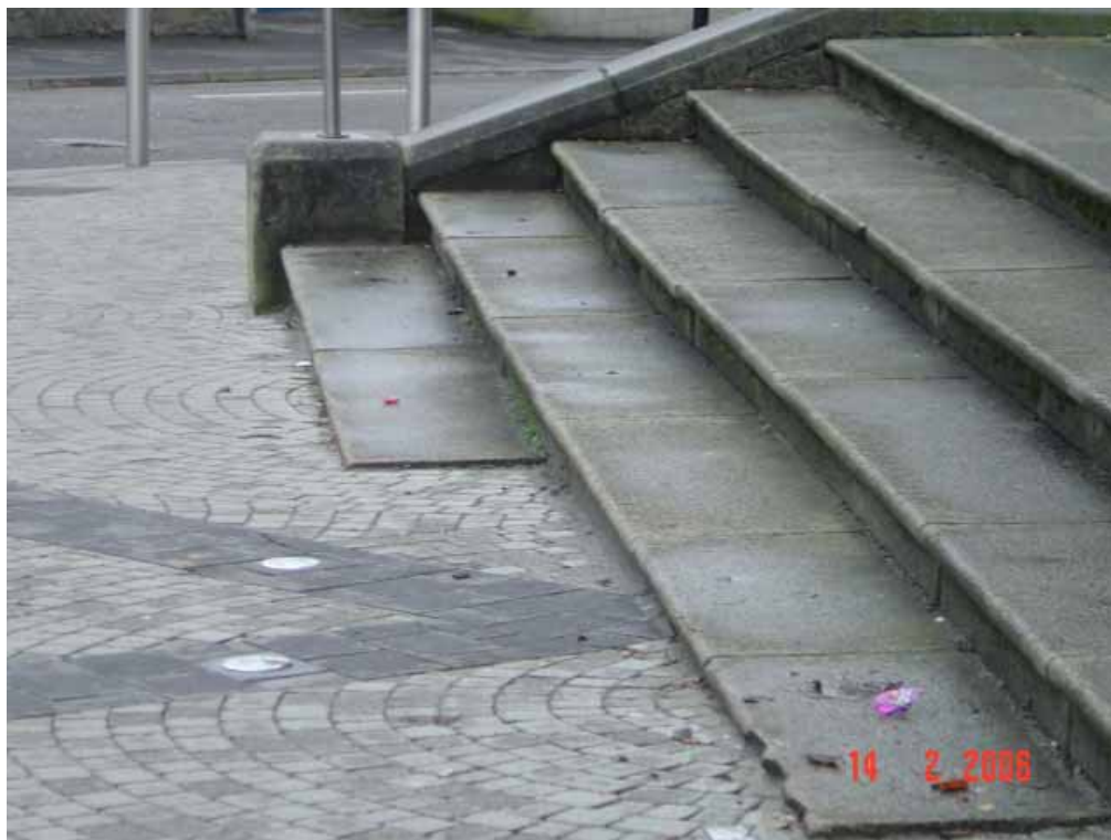
Fig 7.2 These steps have no tactile hazard strips plus the steps have no visual contrasting from the surrounding area.
