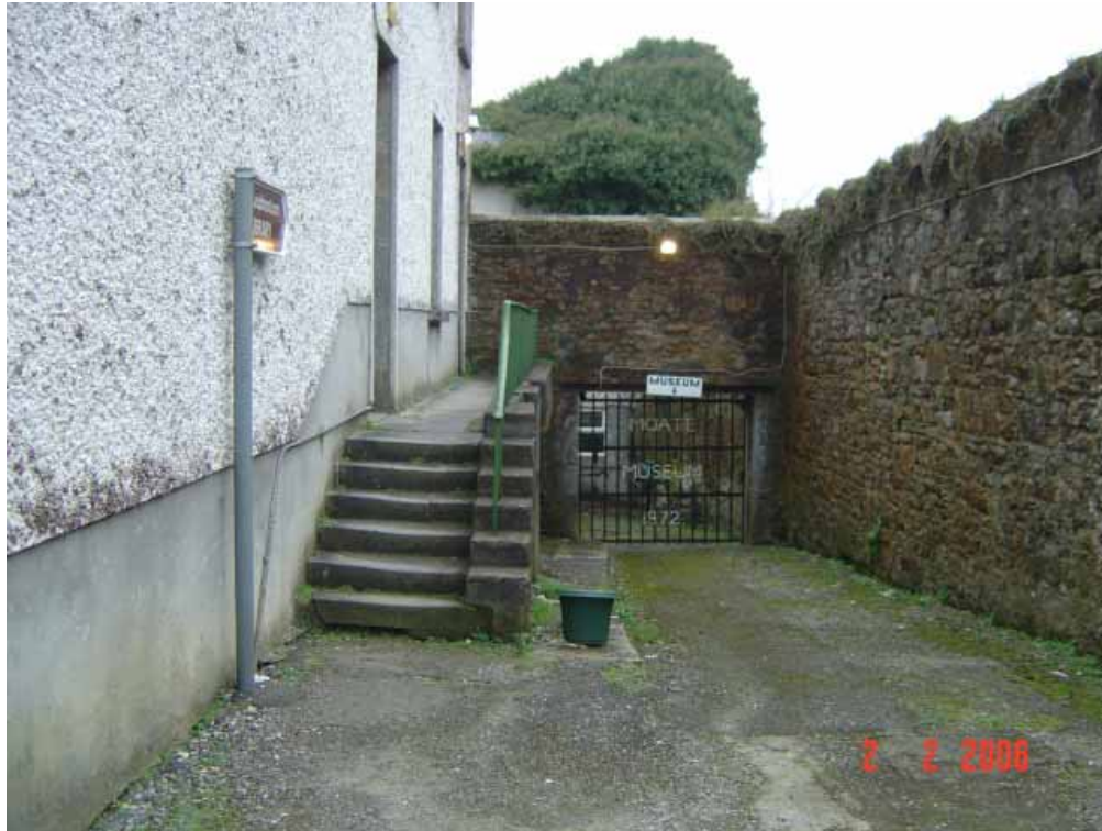
Fig 8.3 Existing steps at entrance.
