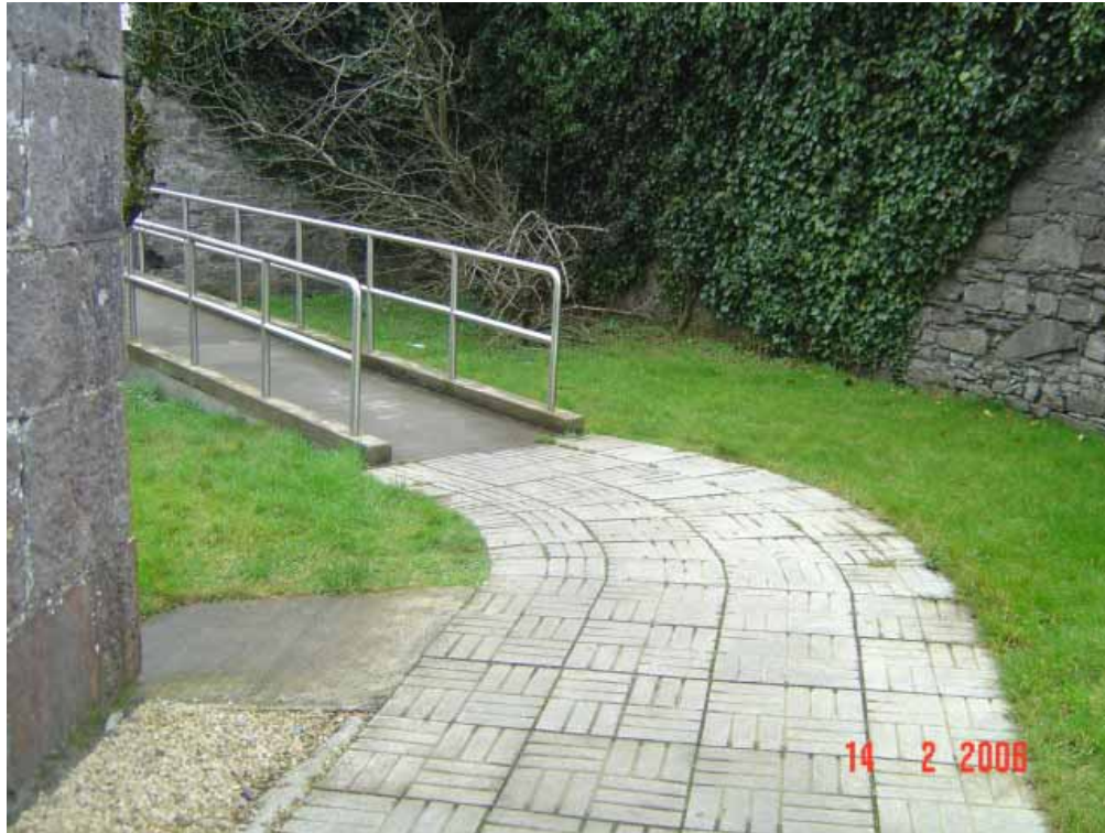
Fig 11.1 Good path leading to ramp but no tactile hazard warning strips in place.
