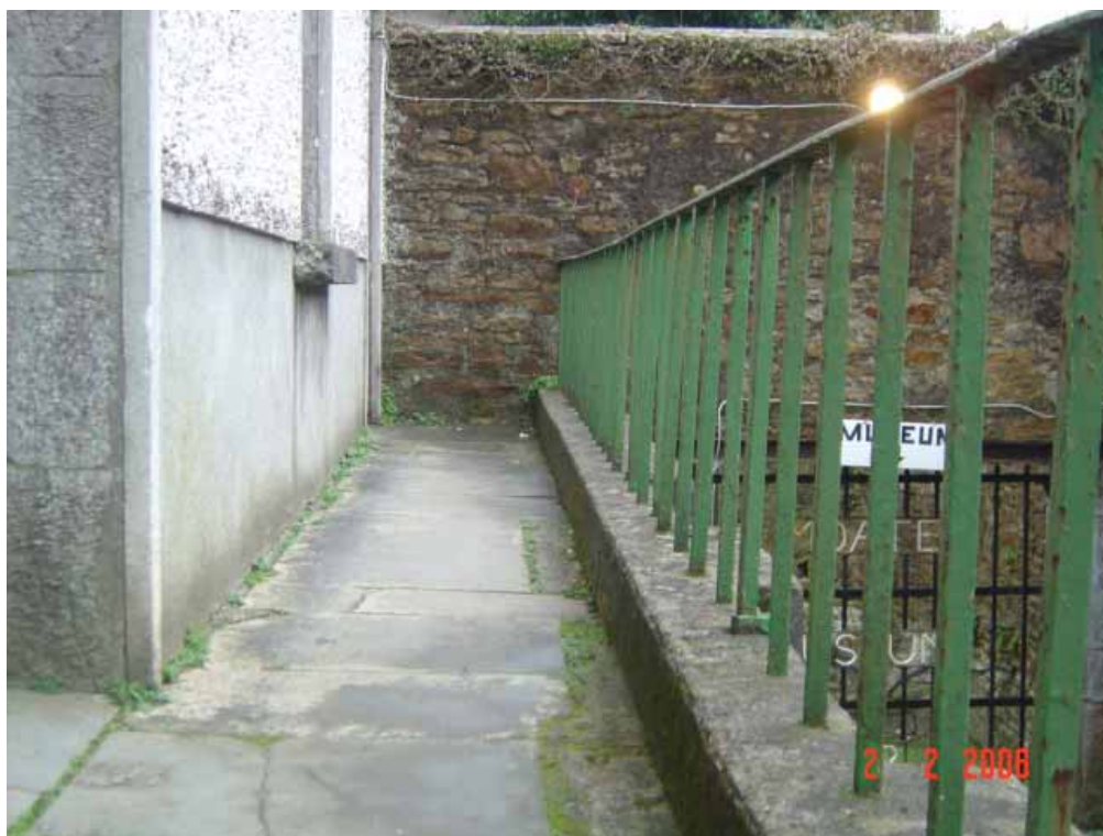
Fig 8.4 Existing path leading to the library door.
