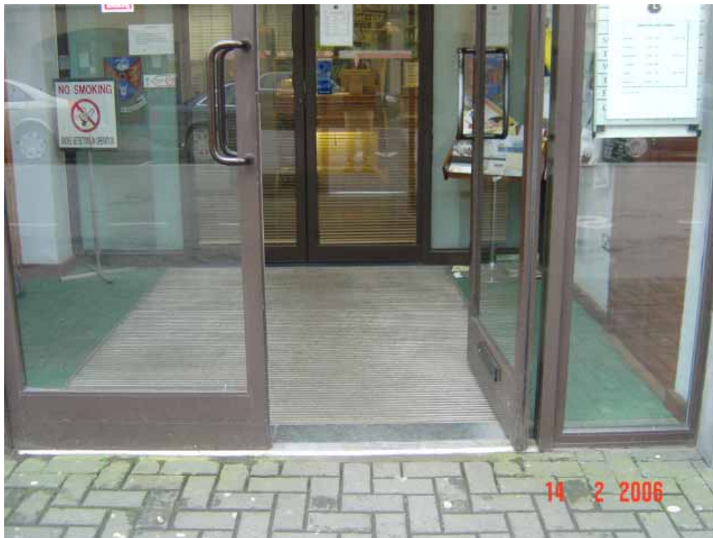
Fig 10.1 Wheelchair friendly access to library with automatic doors on the inside. Entrance needs outside lighting.
