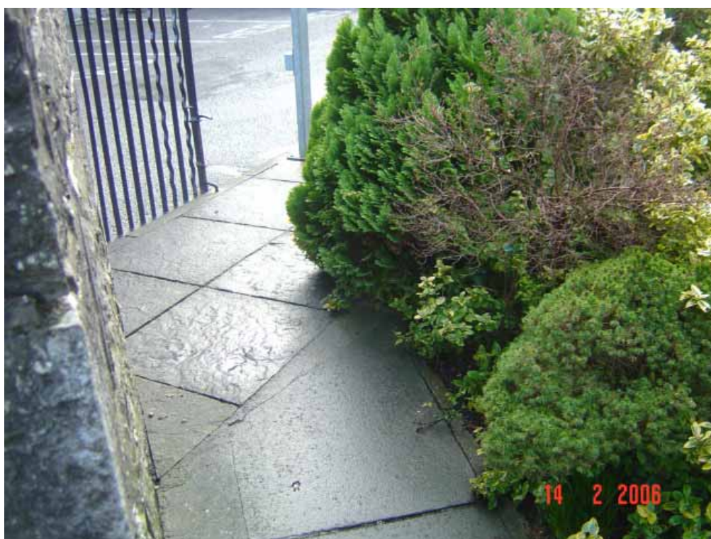
Fig 13.2 Narrow path with vegetation growing over
