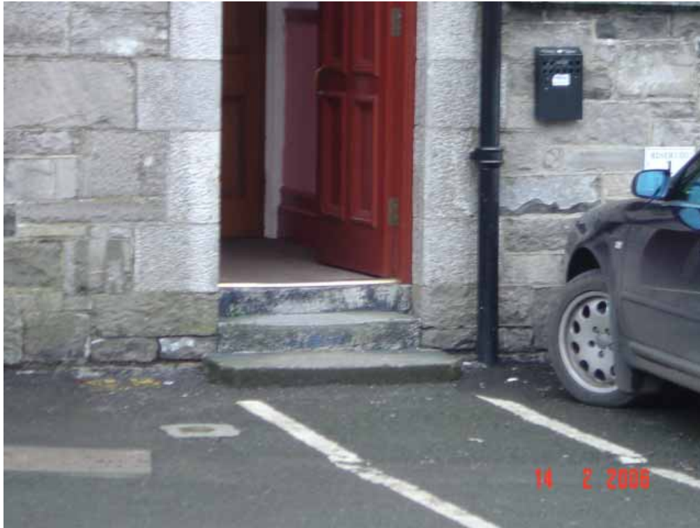
Fig 7.3 These steps have no tactile hazard strips nor are the risers consistent which is dangerous.
